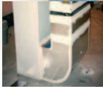
Sealed Ductwork
